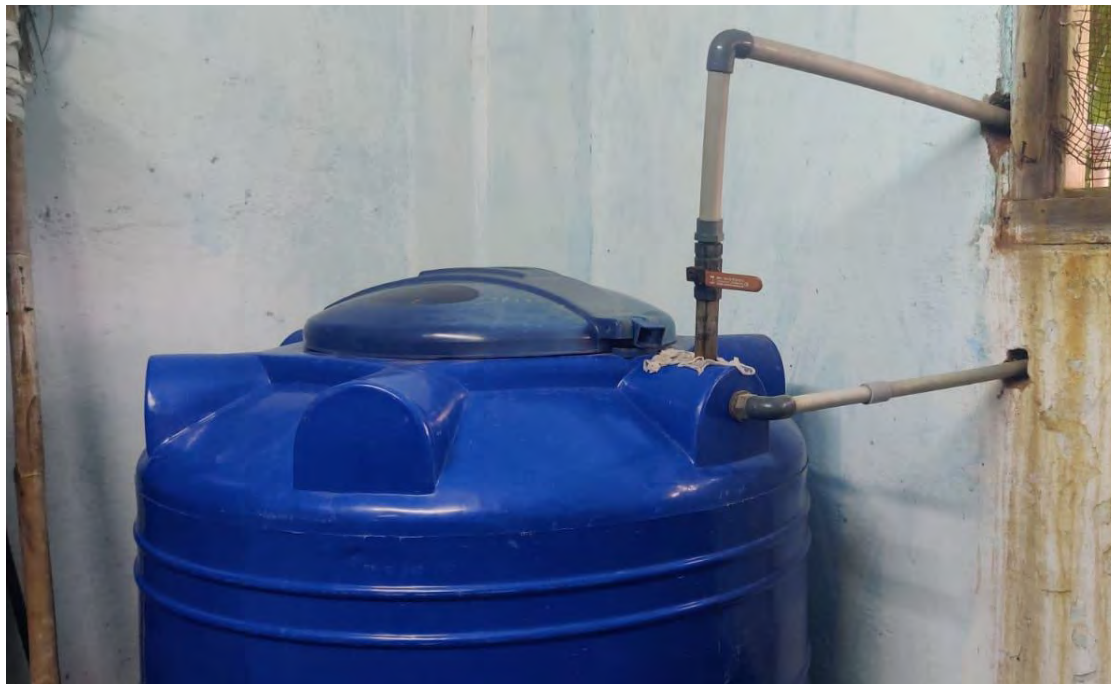
RAIN WATER COLLECTION TANK UNIT TO COLLECT DISTILLED WATER FOR LABORATORY USE (RAIN WATER COLLECTION)
