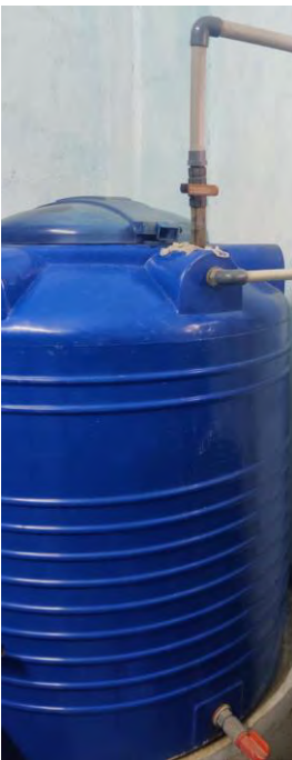
RAIN WATER COLLECTION TANK UNIT TO COLLECT DISTILLED WATER FOR LABORATORY USE (RAIN WATER COLLECTION)
